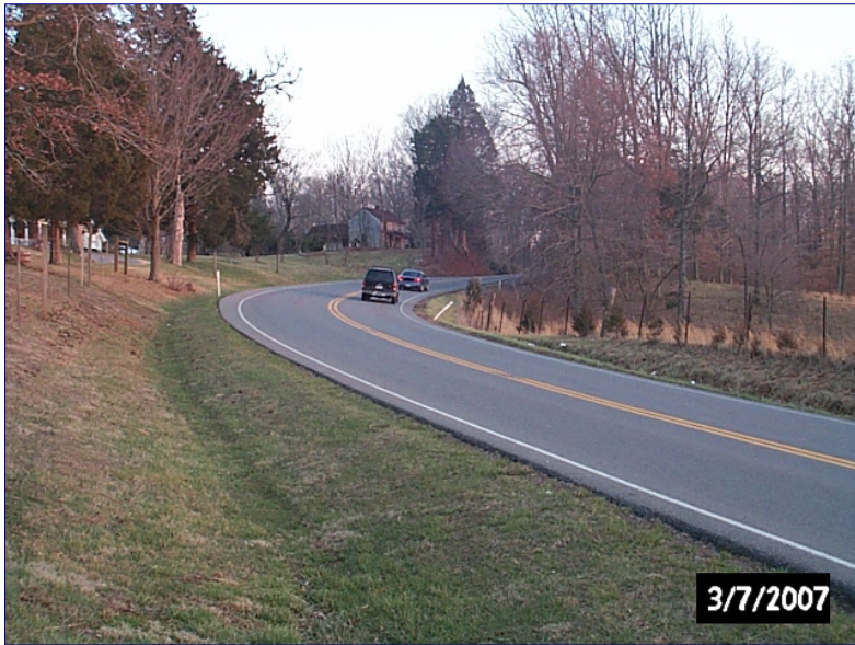
Photo 4 KY 163 south of proposed Tompkinsville Bypass intersection
