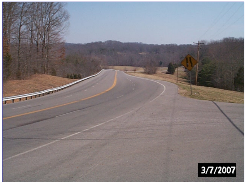
Photo 17 KY 163, 4 Lane Section Near Reed-Ford Road
