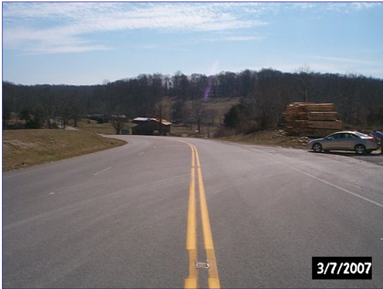
Photo 10 KY 163 at Lumberyard, Looking South
