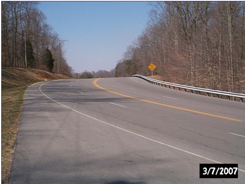
Photo 16 KY 163, 4 Lane Section Near Reed-Ford Road
