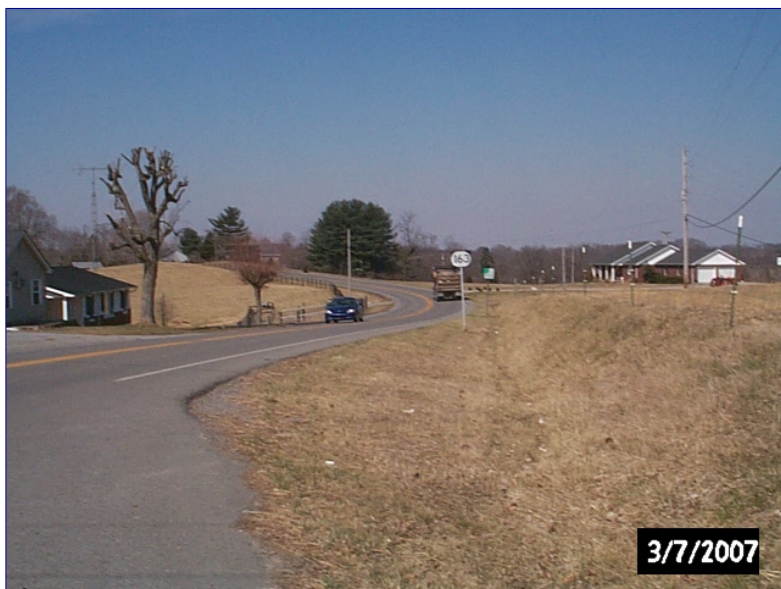
Photo 6 KY 163 at KY 3144, Looking North
