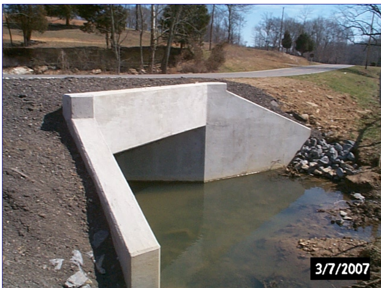
Photo 12 New Culvert at the site of Moore's Mill near Hestand
